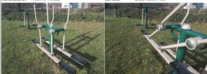
Finding: The swinging movement of the item exceeds the maximum 55 degrees from the vertical required by BS EN 16630
