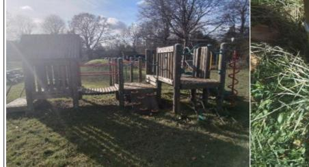
**Finding:** There is some strimmer / machinery damage apparent on the posts, this can penetrate the preservative applied to the timber and accelerate the rotting process
