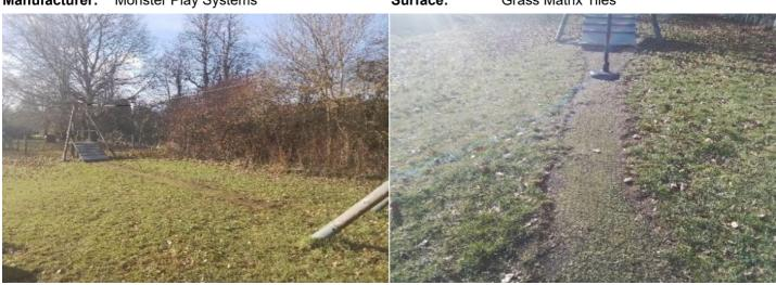
Finding: The grass mats are silted up and the soil is compacted; this may have an effect on the impact absorbing ensure the correct surface qualities are maintained for the properties of the surface
