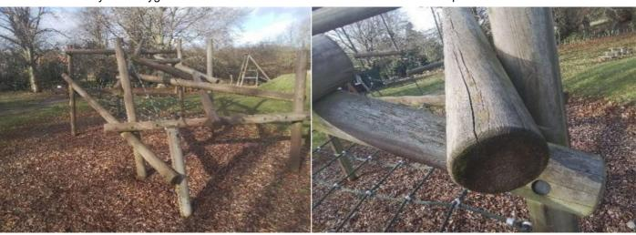
**Finding:** The timber has a number of splits/shakes or air **Action:** Monitor to ensure the splits do not cross through cracks and this may affect the stability or allow water ingress fixing points of the structure and/or cause any instability which will accelerate the rotting process
