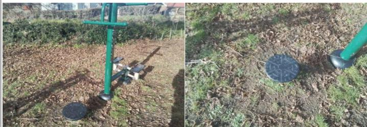
**Finding:** The deflection of the rotating user station exceeds **Action:** Monitor - No remedial work recommended the maximum 105 degrees required by BS EN 16630
