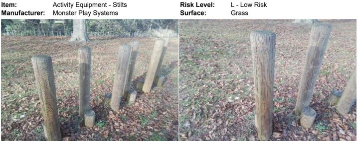
Finding: The timber has a number of splits/shakes or air Action: Monitor to ensure the splits do not cross through cracks and this may affect the stability or allow water ingress fixing points of the structure and/or cause any instability which will accelerate the rotting process
