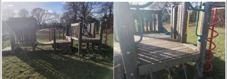
Finding: There is an opening in the barriers exceeding the Action: Monitor - No remedial work recommended width allowed (500mm) in BS EN 1176, this is a low risk failure and no remedial action is required
