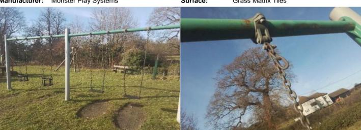
Finding: The chain links are worn in excess of 40% and require renewing
