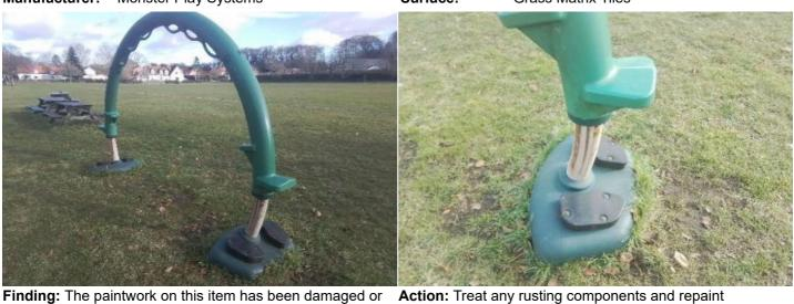
worn exposing the metal underneath which is rusting
